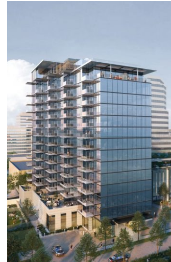
8111 Douglas Avenue Location: Dallas, TX Developer: Lincoln Properties Number of Units: 128 Scope of Work: Kitchen, Bathrooms, Closets Status: In Progress
