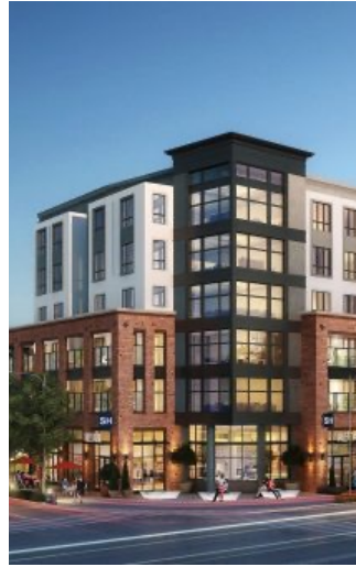
988 EL CAMINO REAL Location: San Francisco, CA Developer: SummerHill Number of Units: 172 Scope of Work: Kitchen, Bathrooms Status: In Progress
