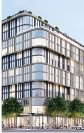
950 SOUTH CAPITAL Location: Washington DC Developer: Related NY Number of Units: 384 Scope of Work: Kitchen, Bathrooms Status: In Progress
